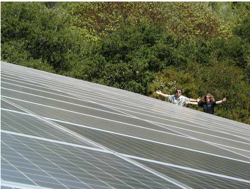
Figure 6.6. Two solar warriors enjoying their photovoltaic system, which powers their electric cars and home. The array of 120 panels ( 300\text{ W} each, 2.2\text{ m}^2 each) has an area of 268\text{ m}^2 , a peak output (allowing for losses in DC-to-AC conversion) of 30.5 kW, and an average output – in California, near Santa Cruz – of 5 kW ( 19\text{ W/m}^2 ). Photo kindly provided by Kenneth Adelman.
