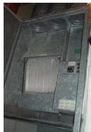
Figure E.11. The Heatkeeper's heat-exchanger.
