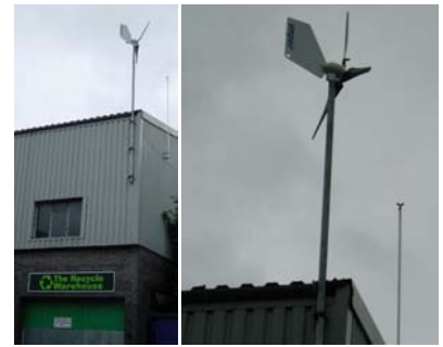
Figure B.9. An Ampair “600 W” micro-turbine. The average power generated by this micro-turbine in Leamington Spa is 0.037 kWh per day (1.5 W).
