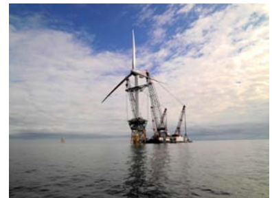
Figure 10.8. Construction of the Beatrice demonstrator deep offshore windfarm. Photos kindly provided by Talisman Energy (UK) Limited.
