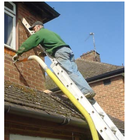
Figure 21.5. Cavity-wall insulation going in.
