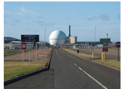
Figure 24.5. Dounreay Nuclear Power Development Establishment, whose primary purpose was the development of fast breeder reactor technology. Photo by John Mullen.
