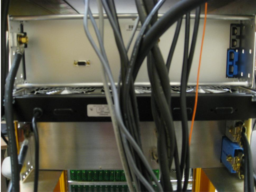
Figure 18. Rear view of two PDBs in the test rack. There are two ground connections (on left) and one of every other connection.
