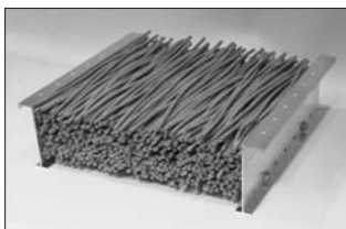
"50%" Fill Per NEC Cross Sectional Area Calculation
